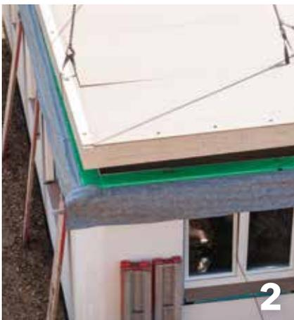
cladding during the lifting, transport and construction stages. Ultrasonic, air leakage testing and thermal imaging can be used to benchmark panel or module performance in the factory and at the finished construction phase. Benchmarking the performance facilitates the assessment of any deterioration during the transportation and installation processes and also proves conformance with the requirements of building regulations.
