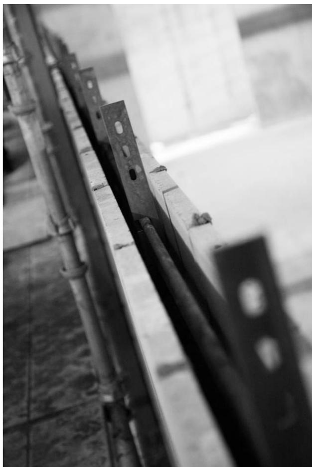
**Figure 1 Exposed WI Beam components ready for concrete installation.
