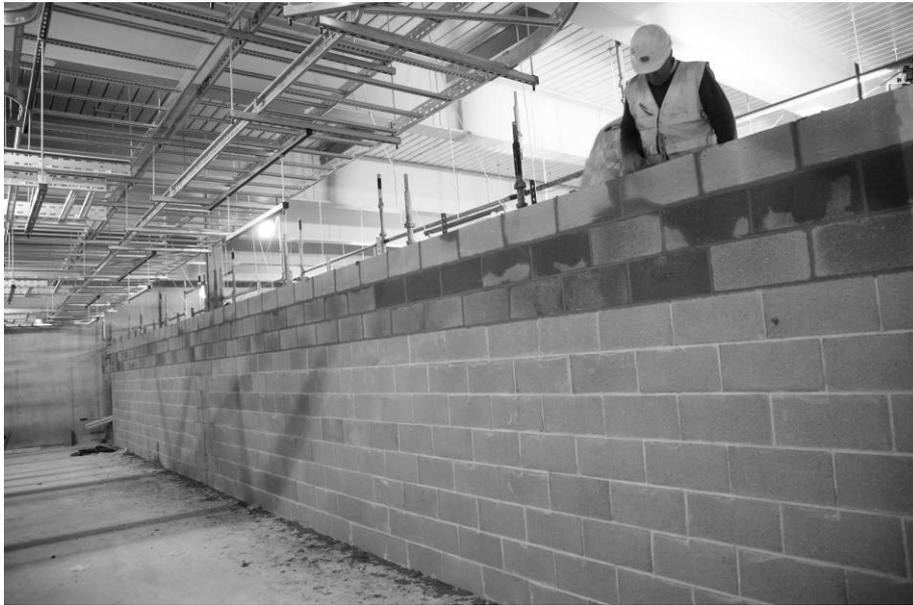
**Figure 2 Construction of an internal WI Beam wall between structural steel columns. The blockwork panel was 9 metres in length and 6 metres in height, and spanned between structural steel columns**
